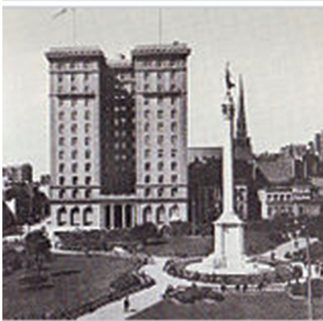
The St. Francis Hotel soon after its opening in 1904 Source: Wikipeda
